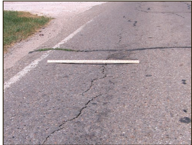
Figure 21. Longitudinal cracks at the bottom of rutting are often caused by structural failure of the subbase.
