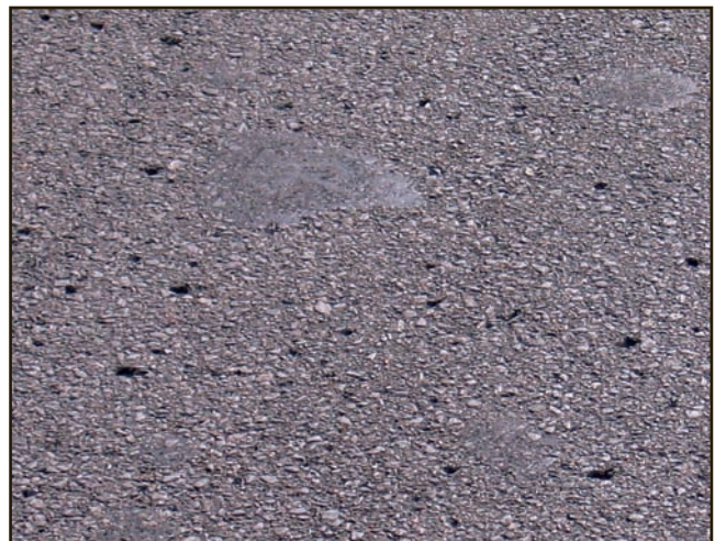
Figure 17. Pocking occurs when pieces of aggregate become dislodge or deteriorate prematurely.
