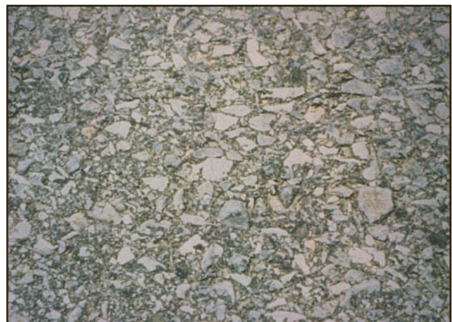
Figure 18. Polished aggregate is smooth pavement with little or no friction. (FHWA)
