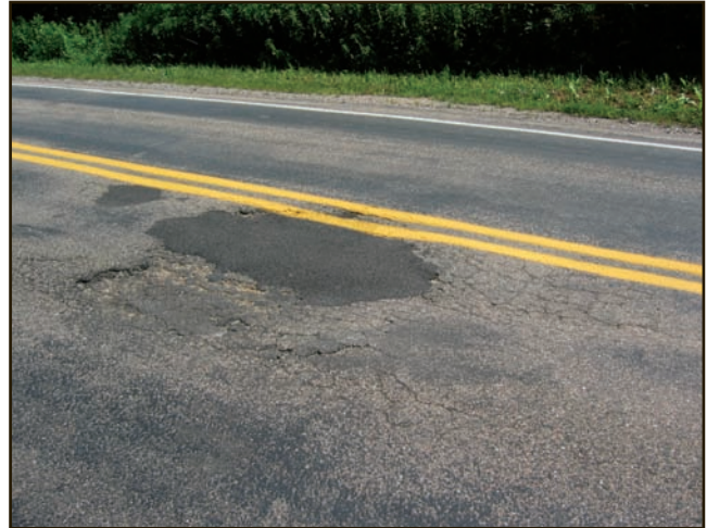
Figure 16. Medium ratings of patching are areas moderately deteriorated that had been replaced with new material.
