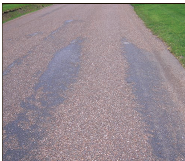
Figure 25. High severity raveling of a seal coat.
