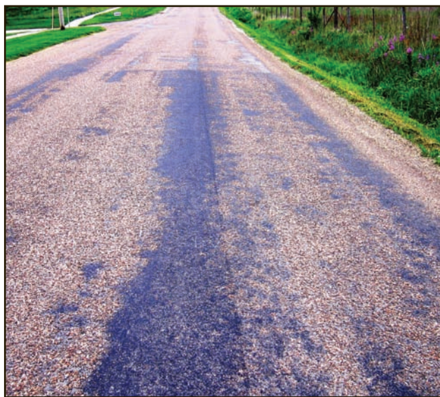
Figure 26. New raveling of a pavement surface.
